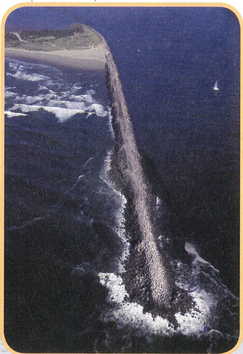
▲ People build jetties, like this one at Coos Bay, Oregon, to stop the loss of sand from beaches.
